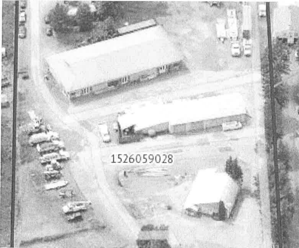
2017 Aerial – shows structural changes to west building. Changed garage doors to man doors, previous man doors and windows have been removed
