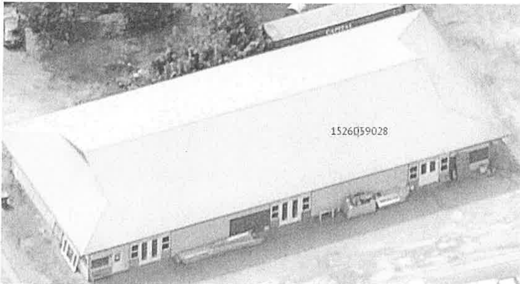
2017 close up of west building
